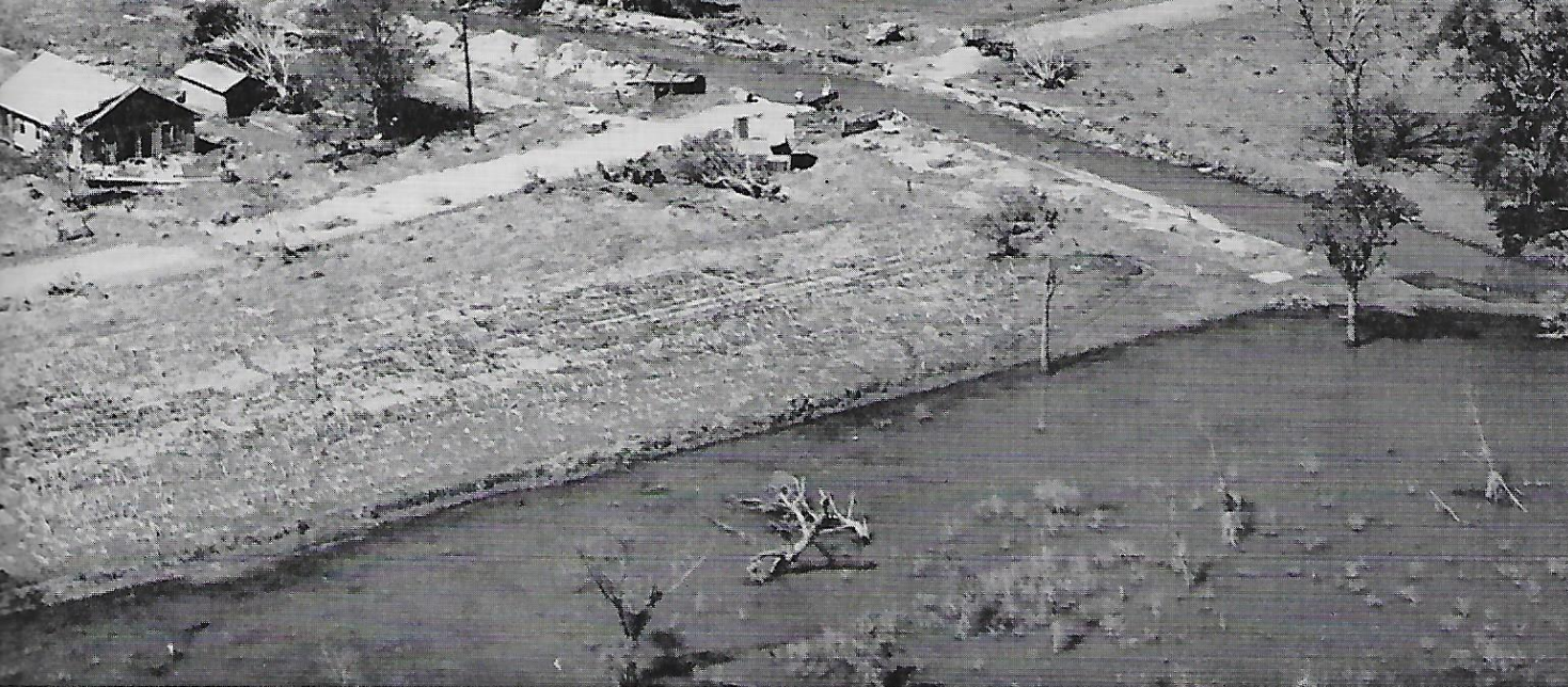
A 10-foot wide drainage ditch, center, that once crossed the island was widened by the hurricane and wave into a canal 60 feet wide.
